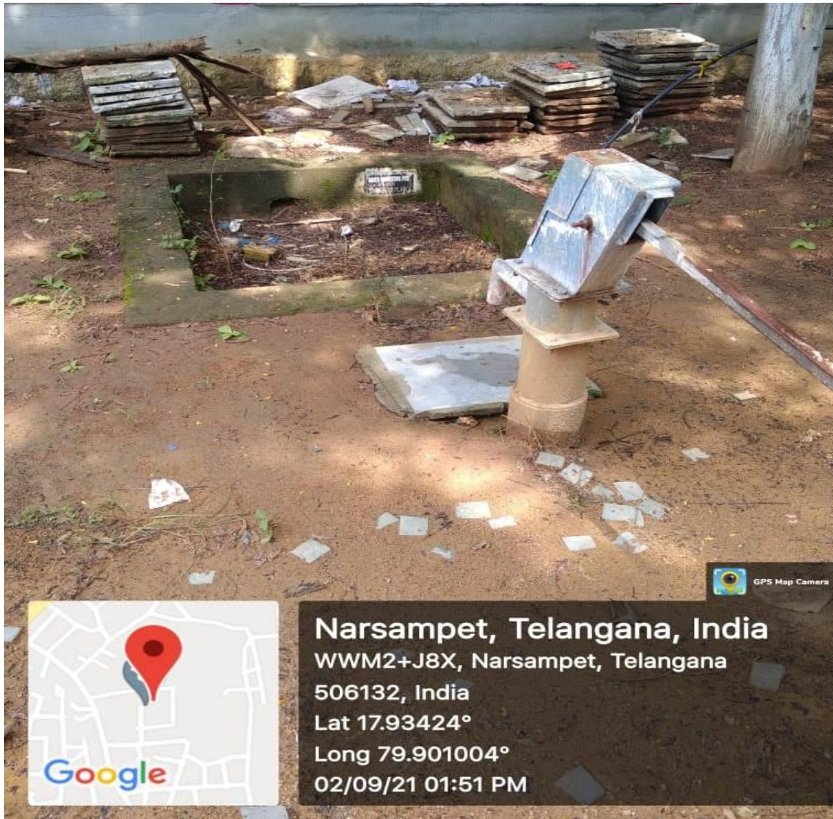
Water harvesting /Recharging pit was dug near the Hand pump
