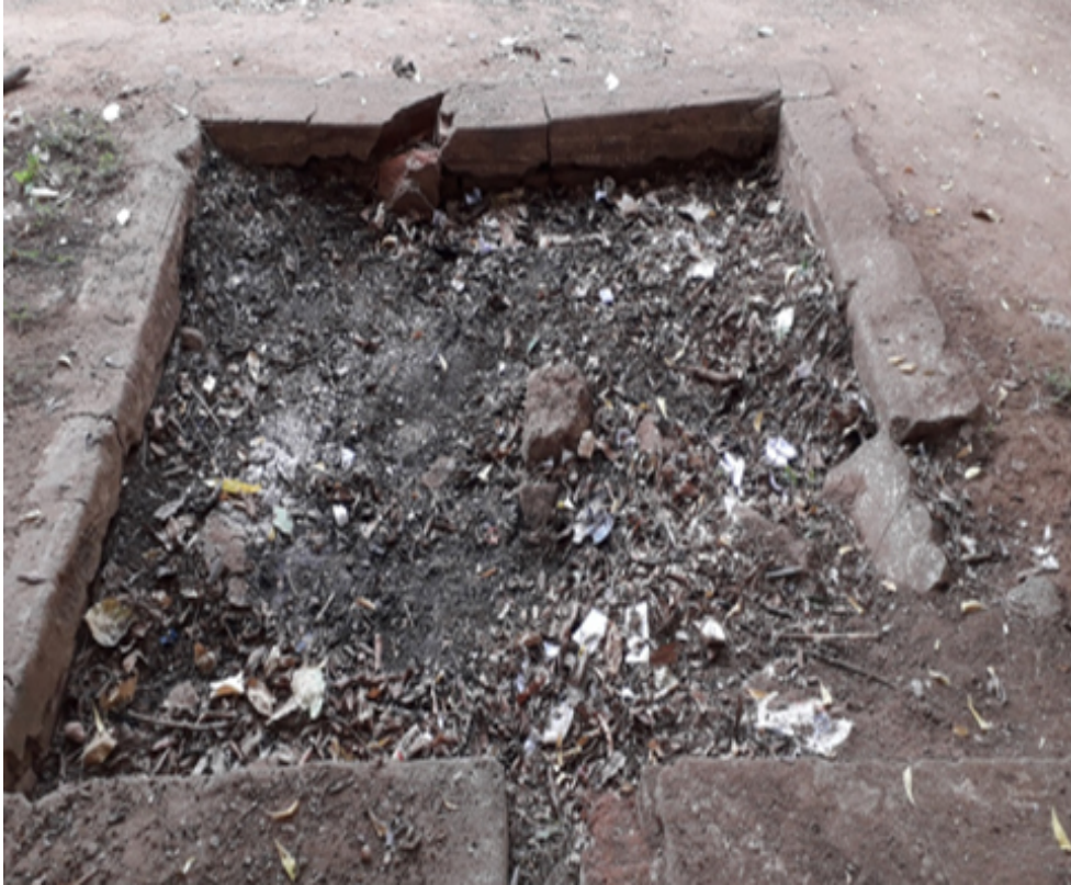
Soaking pit under repair
