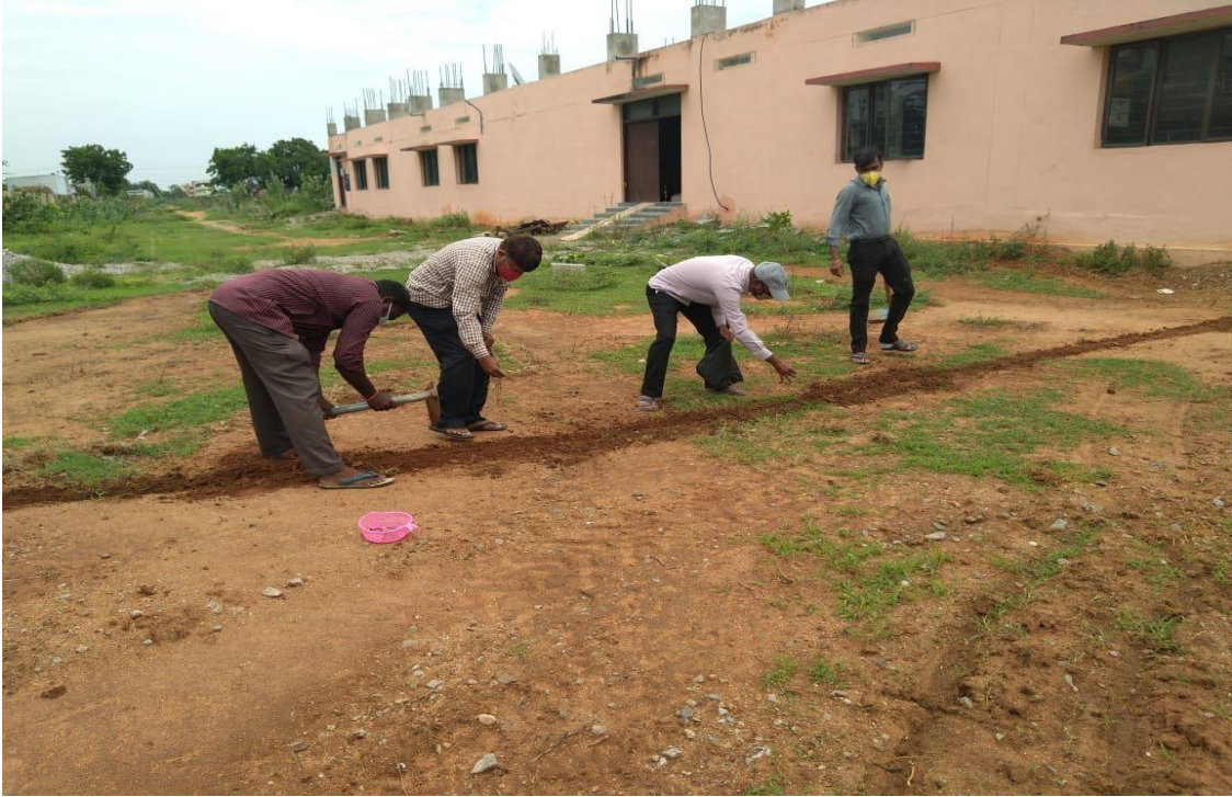
Chanalising waste water
