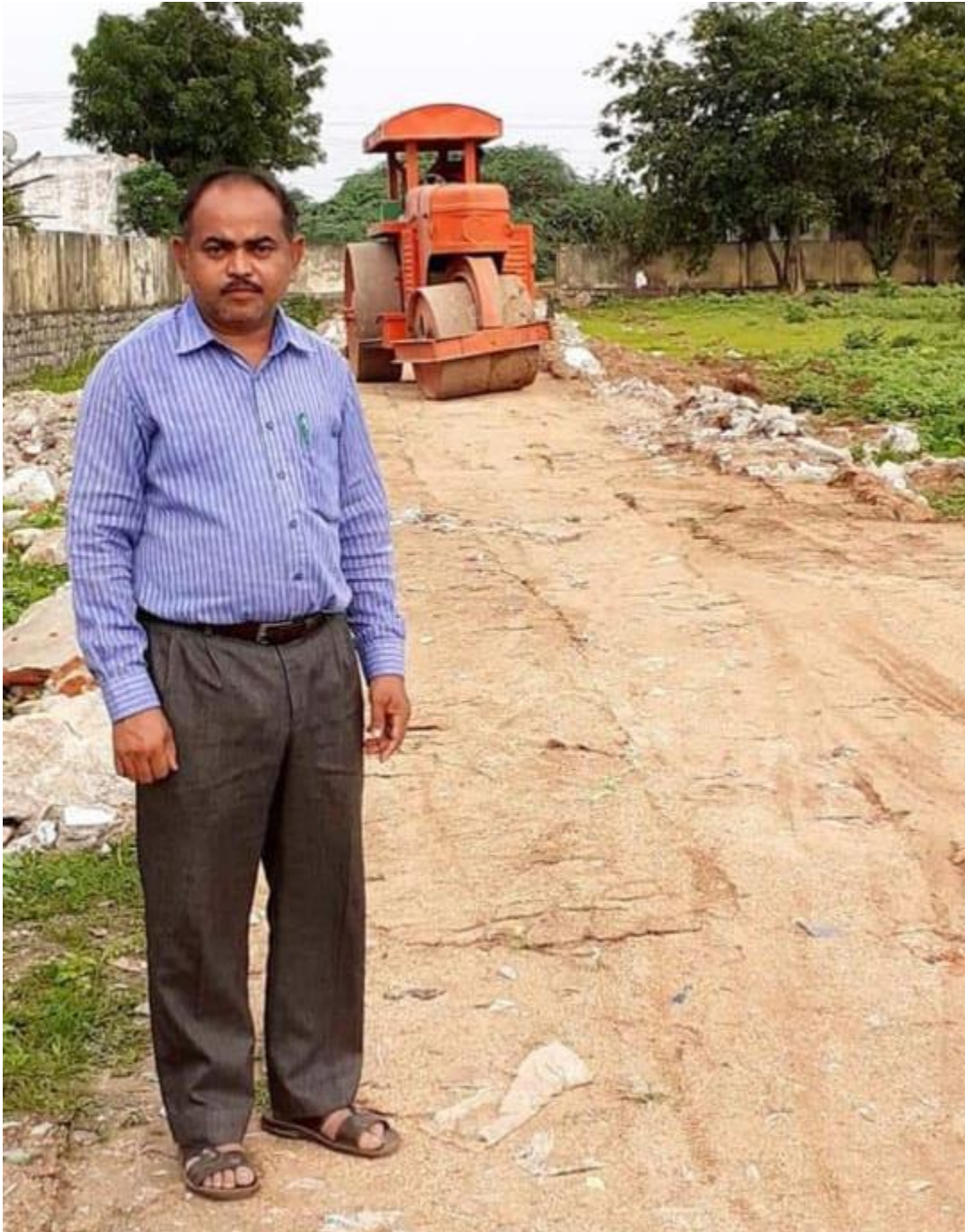
Working on pathway formation
