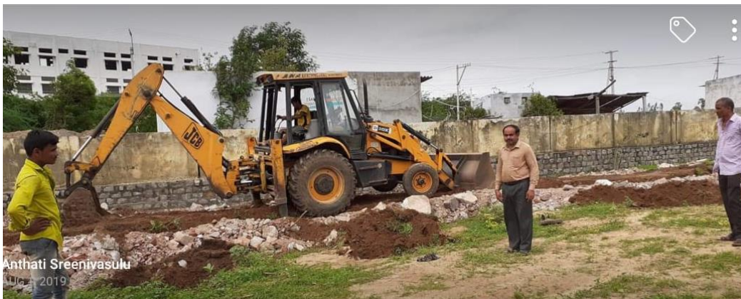
Working on pathway formation
