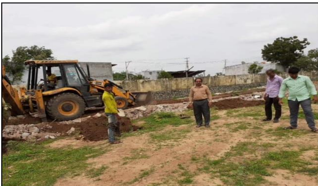
Working on pathway formation
